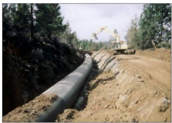
Beginning in 2000, three phases of the project have been completed resulting in the installation of over 10,000 feet of 84" RSC 213 Weholite pipe with additional earth ditch replacement sections under consideration.
